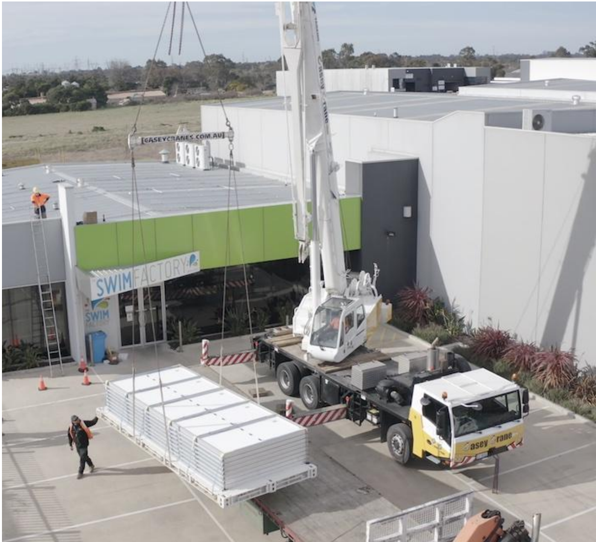
Example of lifting a stack of Solpods using chains through the tyne pockets of the pallet
