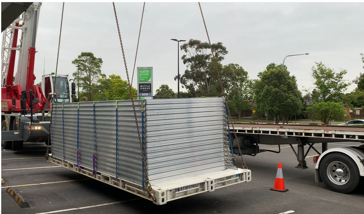
Pallet of Solpods being lifted off truck using a crane, spreader bar, chains, and lugs that connect to the corner castings of the container base.
