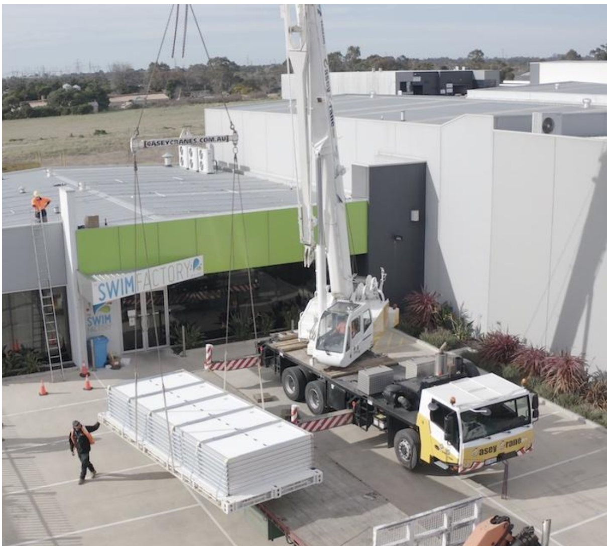
If lifting lugs aren't available, chains can be fed through the tyne pocks.
