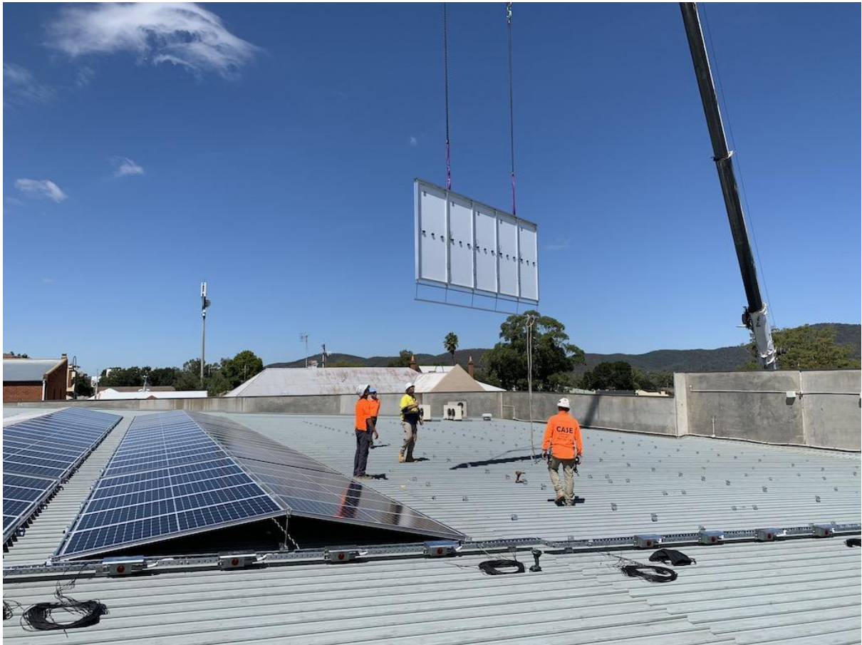
Mobile crane lifting a Solpod to a roof
