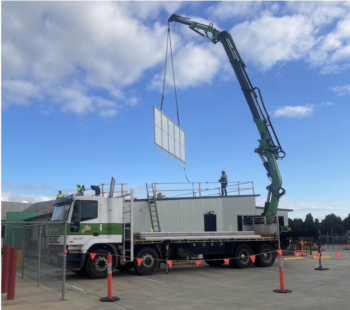
Crane truck lifting Solpods onto a roof.
