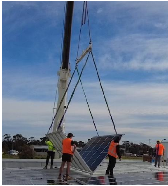
Solpod being lifted to the roof and unfolded using a 3 metre spreader bar and 3 metre chains (or slings) with hooks at the end, to connect to the 1 metre slings that are fixed to the Solpod.
