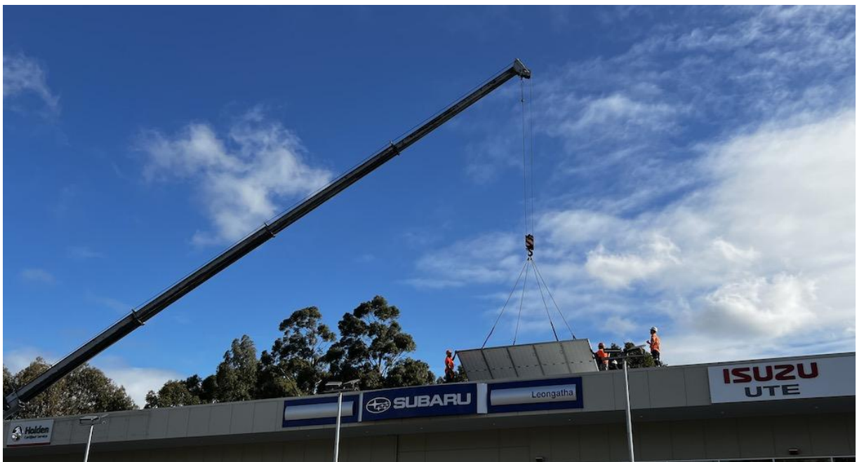
Solpod being lifted and unfolded without a spreader bar. Ideally, use longer chains e.g. 5 metres.
