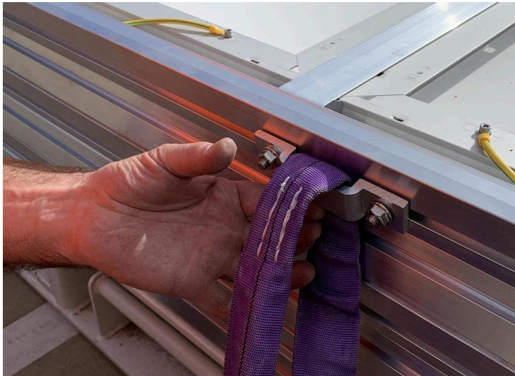
1 metre sling and sling bracket, fasteners about to be tightened
