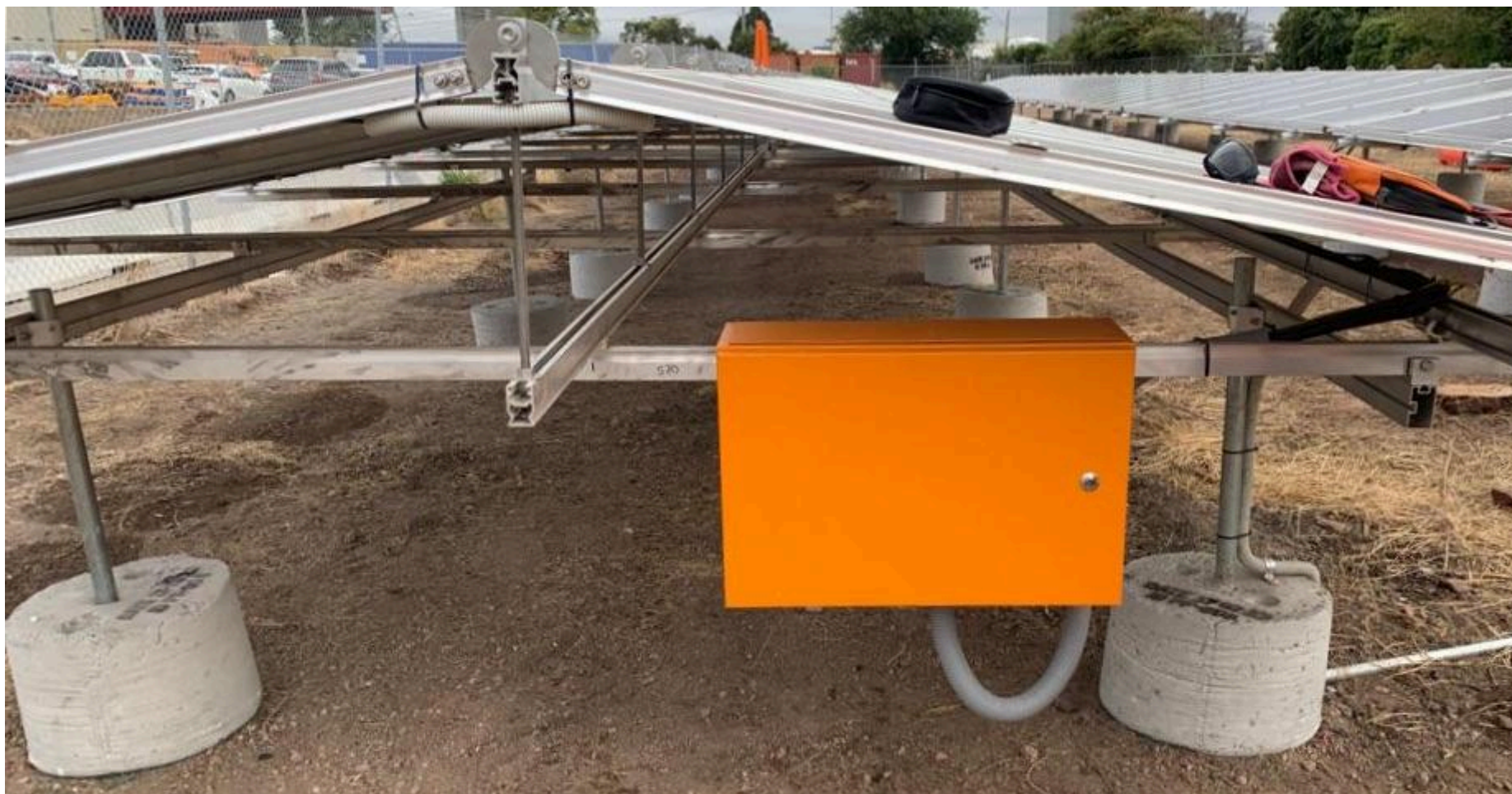
Solpod Channel fixed under Solpods, used to carry DC cables to a termination point
