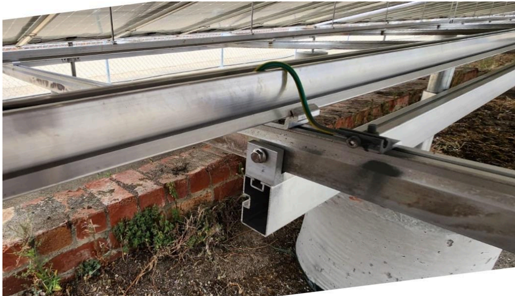
Earth cable attached to earth lug (SPEL-GB37) that fixes to a joist, with zinc spray.
