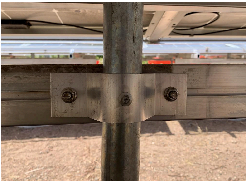
Riser bracket fixed using 12g Tek screw
