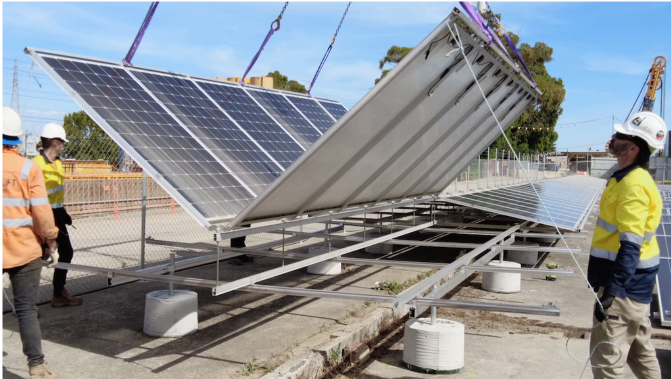
Solpod being unfolded onto a ground frame
