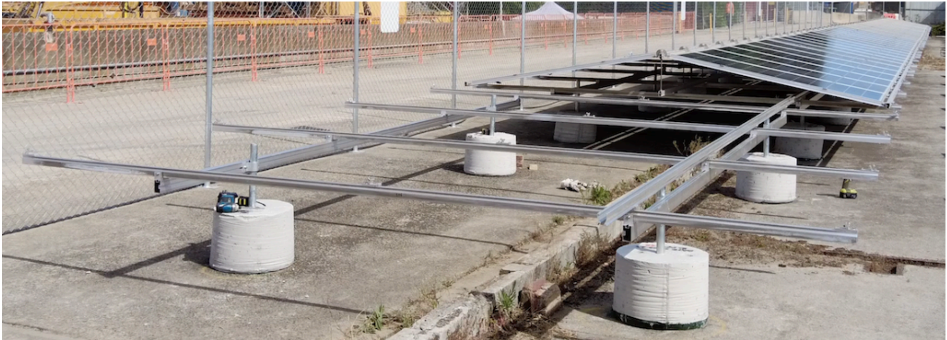
Example installation of Solpod Ground (patent pending)
