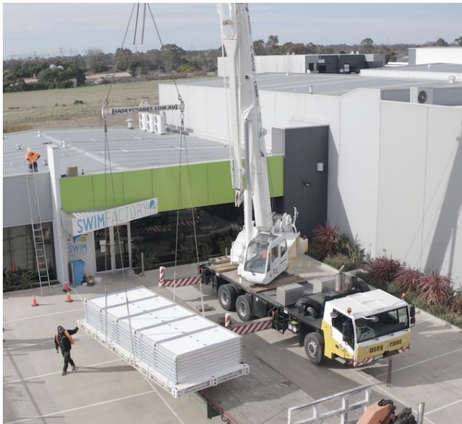
Container base being lifted off truck using a 3 metre spreader bar, hired with crane
