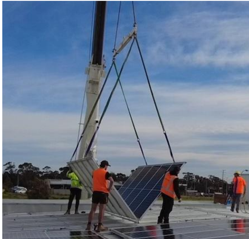
Solpod being unfolded
