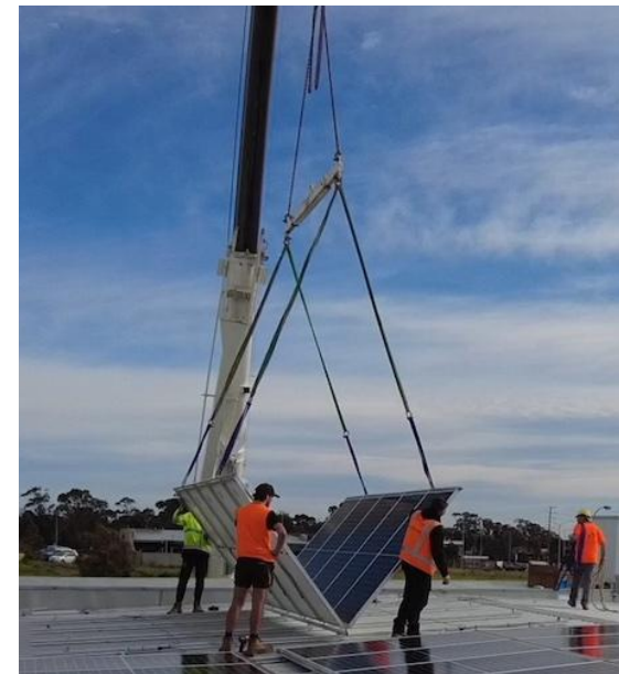
Solpod being unfolded on roof
