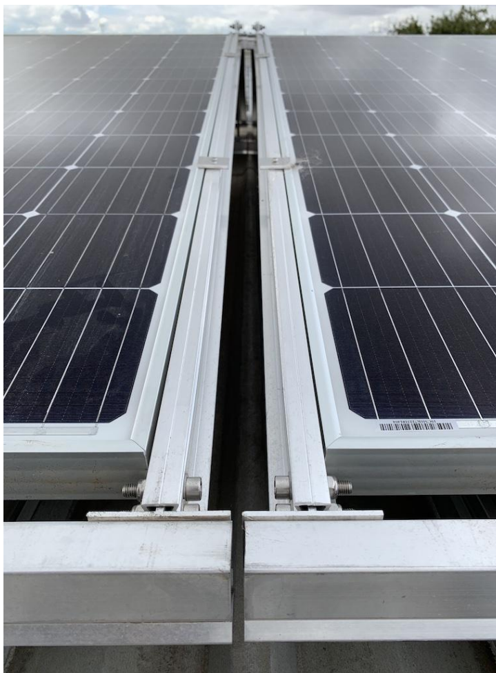
Small gap between Solpods to simplify DC cable connections between Solpods
