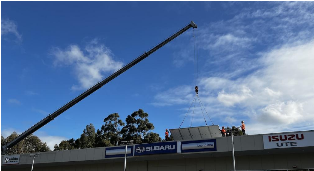
Solpod being lifted and unfolded without a spreader bar
