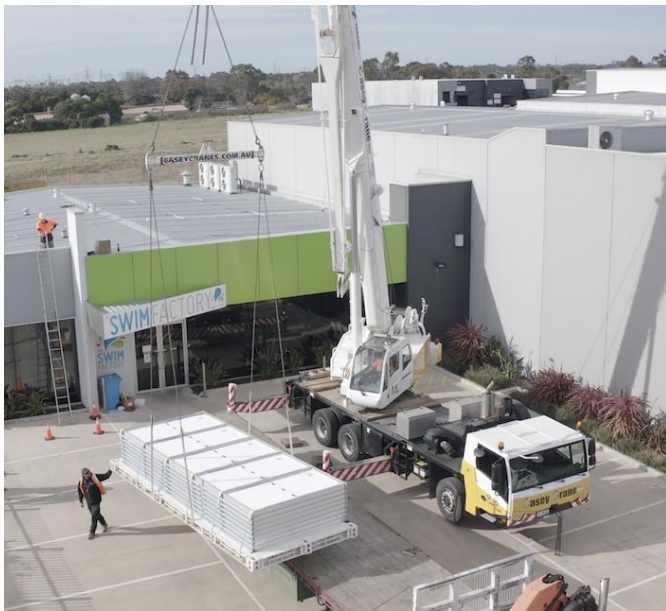
Container base being lifted off truck
